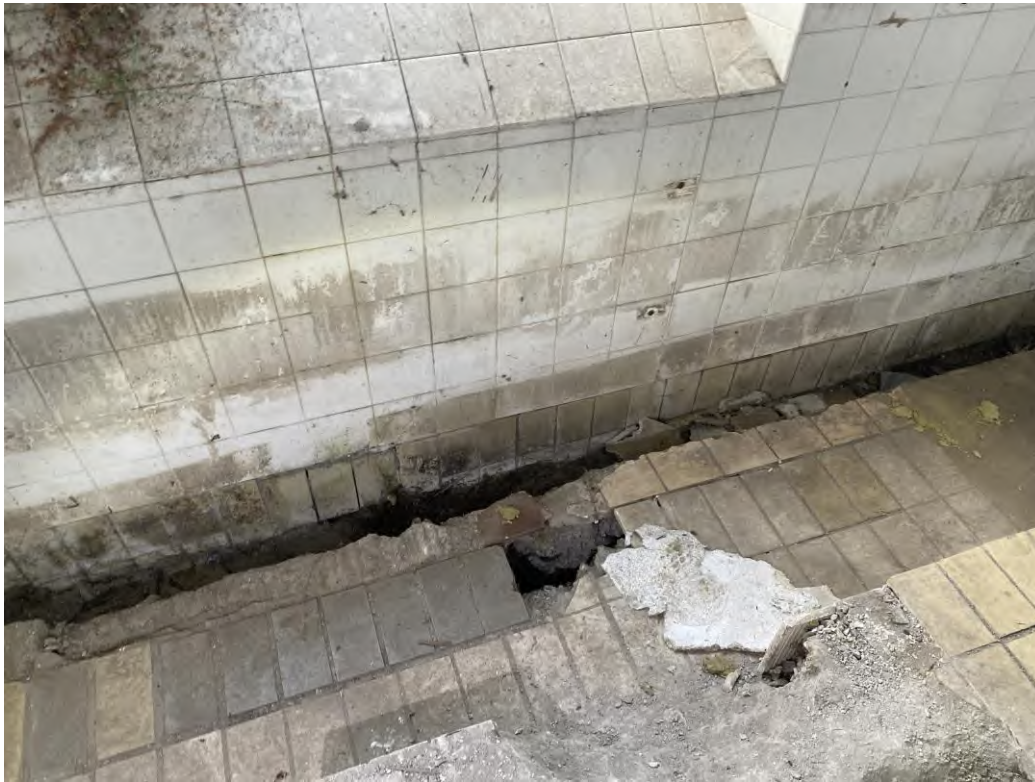
Ceramic floor tiles in building 5
