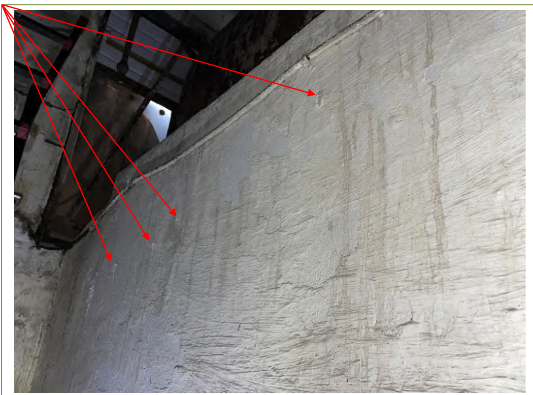
Asbestos containing thermal insulation residue on the walls and pipework in the boiler room
