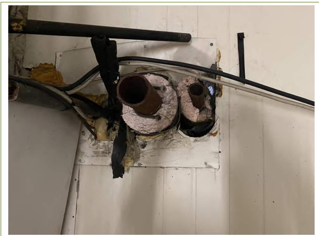
Pipework insulation sampled in building 5
