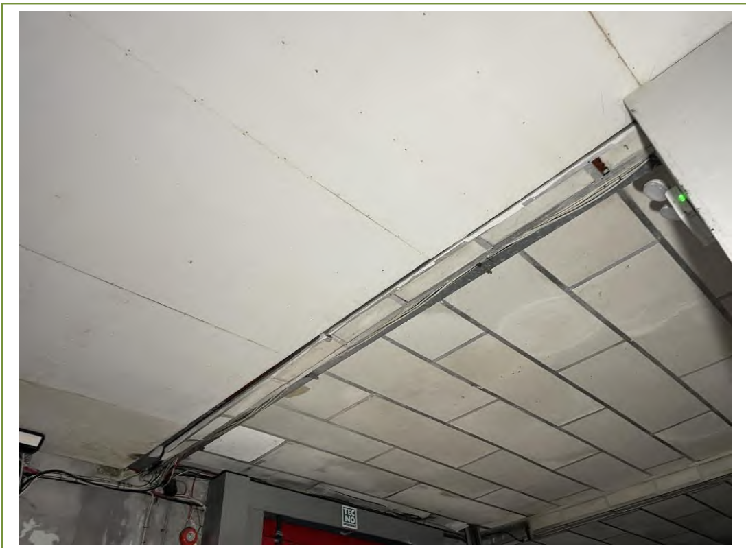
Asbestos insulation board on the ceiling and around the beams in Building 12
