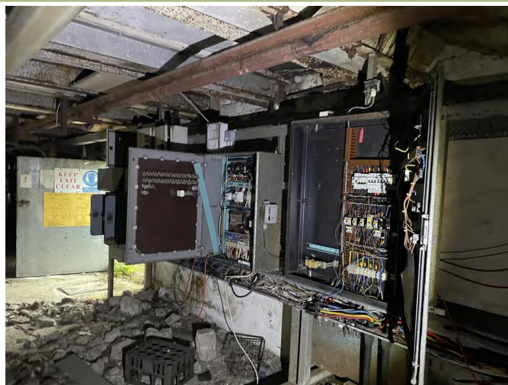
Spark arrestors and backing boards on redundant electrics in building 2
