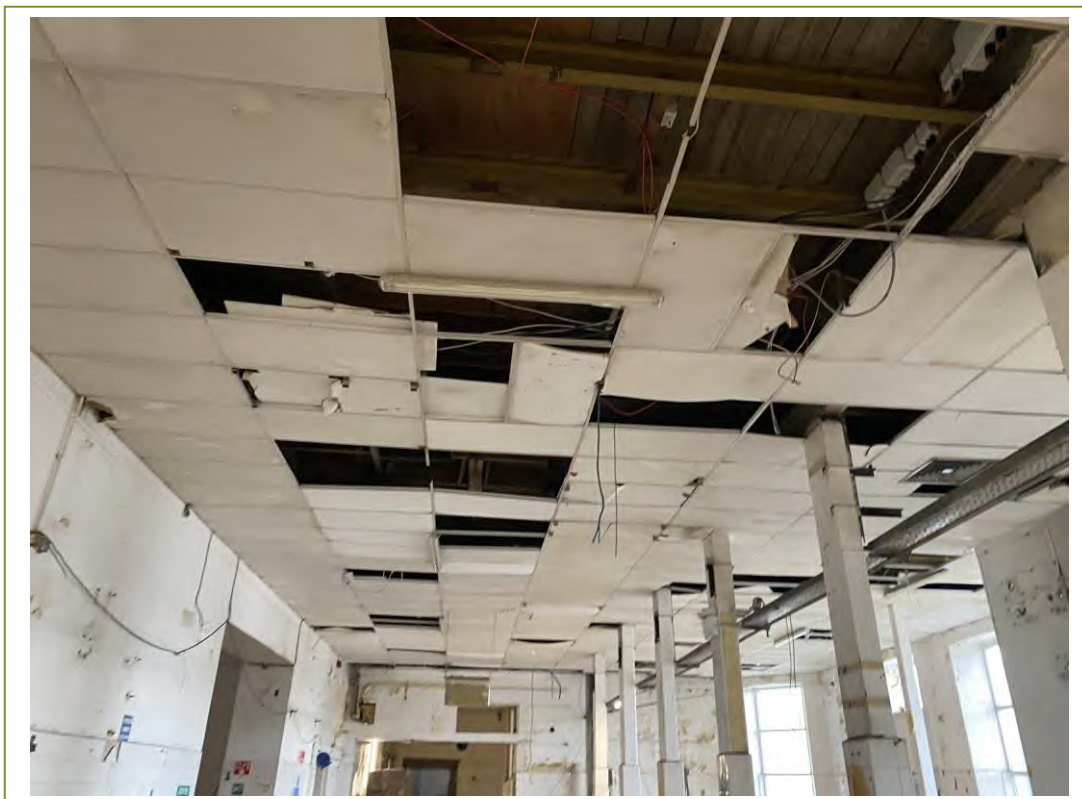
Plasterboard ceiling tiles in building 5
